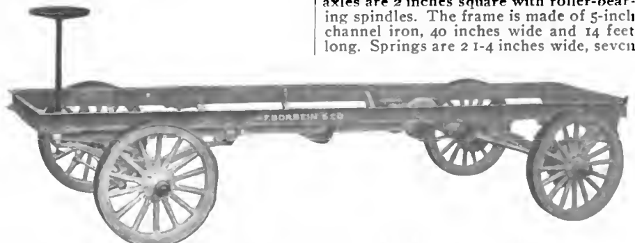
BORBEIN SIDE-CHAIN DRIVE RUNNING GEAR FOR HEAVY TRUCKS.
